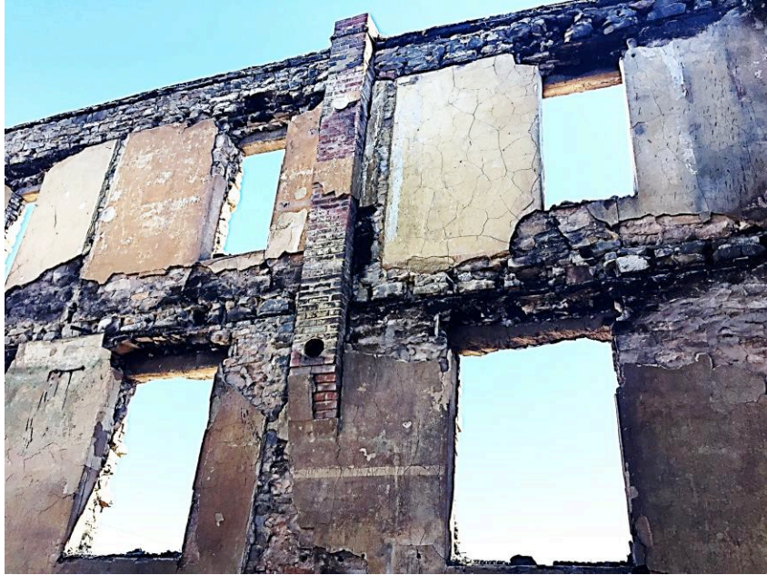
Figure 2. Photo of interior of east wall showing remnants of interior plaster, joist pockets, stove chimney, and burned interior lintels.
