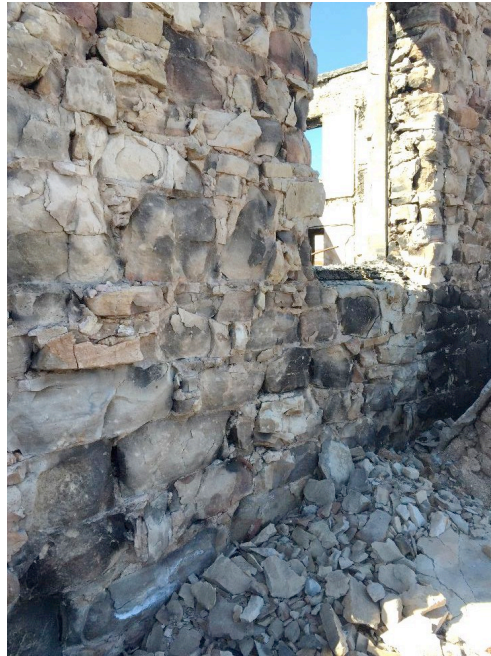
Figure 1. Photograph of exterior of east wall showing delaminated and fallen sandstone. Photo also shows random sizing and bonds of stonework.
