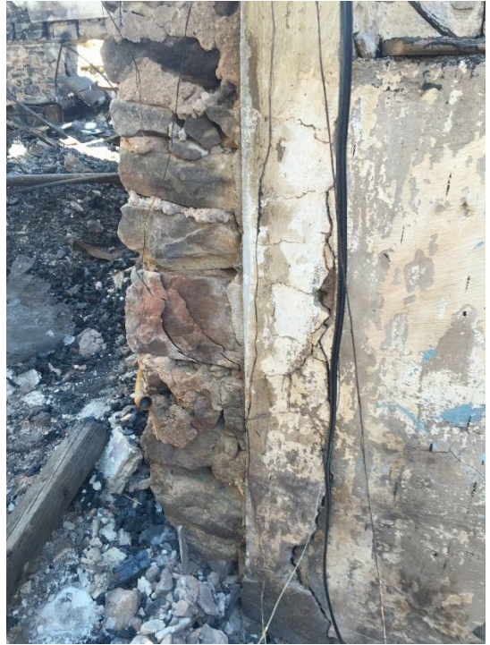
Figure 3. Detail of section through 1 st floor window showing cracked stone and plaster.
