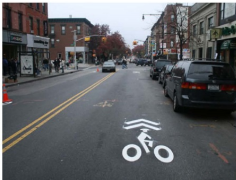
New Pavement and Striping
