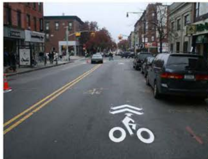
New Pavement and Striping
